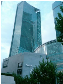
Plaza Tower Shanghai
